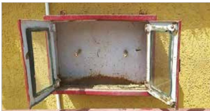
(a) Empty Hose Box - No Hose & Nozzle.
