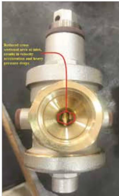
Figure-2: Piston PRV with reduced ports
