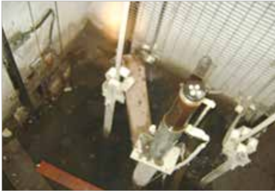
Water in the hoistway pit
