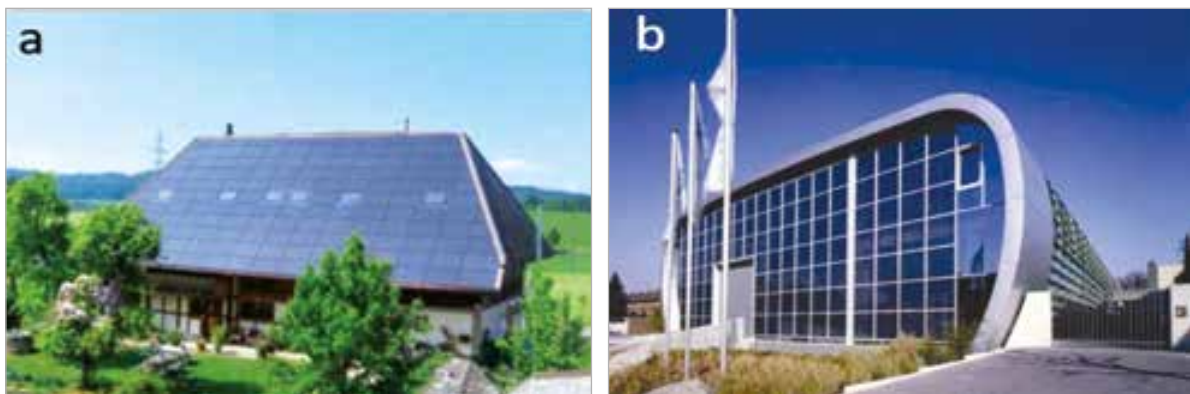
Figure-1: (a.) Umweltarena Spreitenbach (Switzerland 2012): an example of a 203% Plus Energy building achieved by means of a customized 750 kWp full-roof BIPV skin consisting of c-Si panels with an antireflective glass (b.) Ferdinand-Braun-Institute, Berlin: 732 dark CIS modules designed as a curved façade (Surface: 640 m 2 , Energy output 39 kWp)
