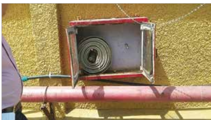
(b) Hose Box - With a Hose but No Nozzle
